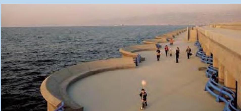
Structures and geometries for reducing the reflection waves.
